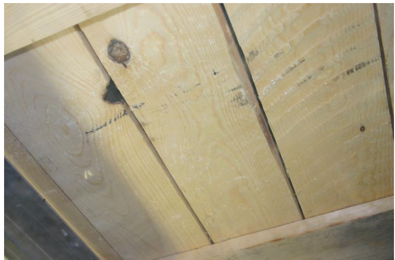
Photo 3 Detail of the substructure of test specimen 1 before testing.
